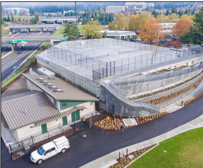
Ridgewood View Park Reservoir
